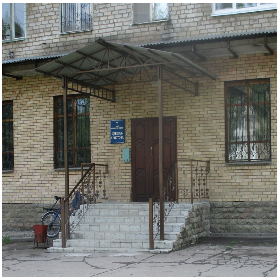
Main entrance to church building in Kramatorsk
