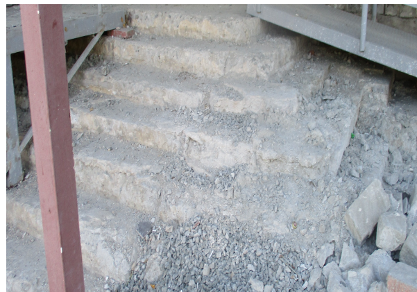
The second entrance steps were in like condition before the repairs.
