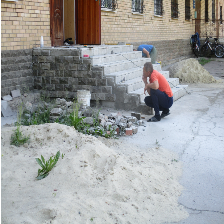
Workman working on second entrance to the building.
